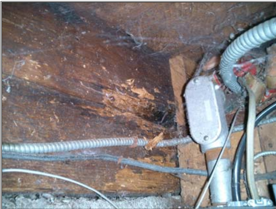
Beetle damage
